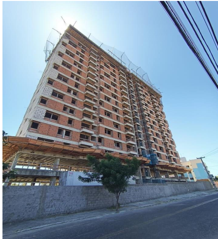
Figura 21 - Obra Volpi Art Residence
