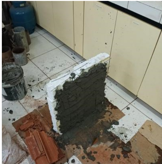
Figura 5 - Reboco do painel de EPS.
