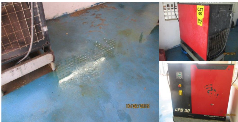
Figura 19 - Compressor Chicago Pneumatic CPB 30
